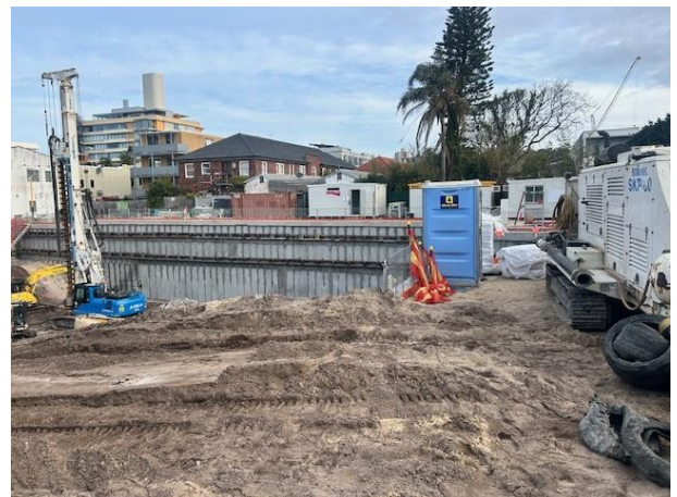
Figure 4: Excavation commenced on site, facing south
