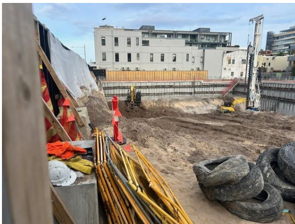
Figure 3: Excavation commenced on site, facing east
